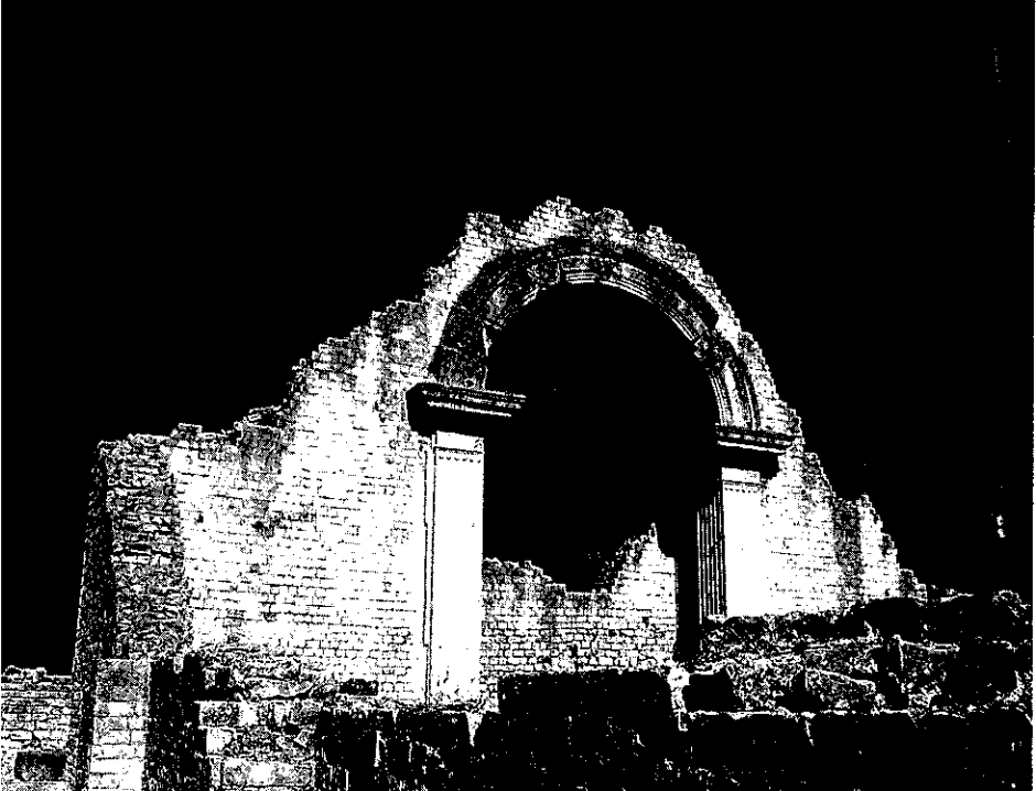
Roman Architecture. This magnificent arch is among the ruins left by the Romans in Vaison-la-Romaine in southern France. The Romans were unsurpassed in their ability to construct elaborate arches, which allowed buildings to carry great structural weight. In this example, the arch rests on columns clearly influenced by Greek architecture.
